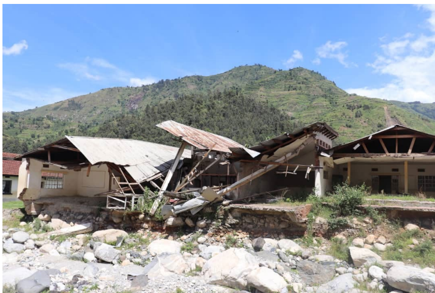
A school destroyed by River Nyamwamba flooding in Kasese District. Photo credit: Elizabeth Nakiru/Oxfam.
